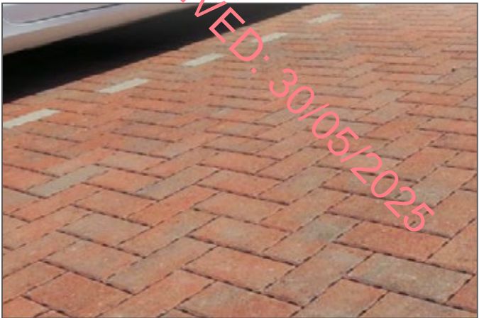
Parking Bay Paving (or similar approved) Kilsaran Clima-Pave Slane - Curragh Gold Size: 200x100x80mm. Herringbone. Border: ClimaPave Newgrange. 3 Size Mix x 80mm in Silver Granite. Soldier Course. (Black granite border for visiotr parking)
