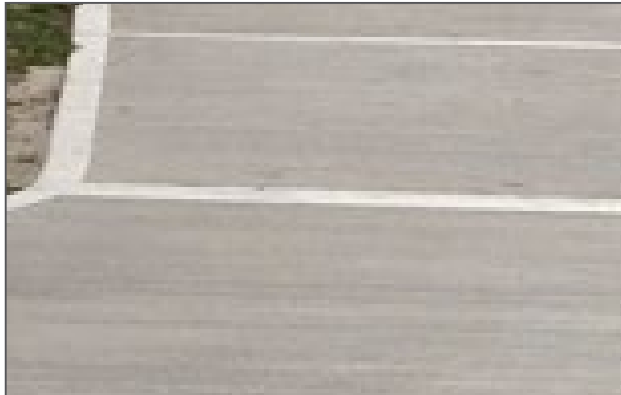
Concrete Footpath (to Engineer's Specification) In-situ concrete. Brushed with trowel edge finish
