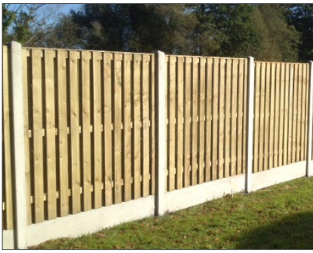
Residential Boundary Fence (1.8m high) Timber Panel Fence with concrete post & gravel board, or similar approved.
