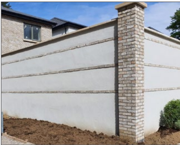
Feature Wall (2m high) Rendered Block wall with brick thread, coping, and piers. or similar approved
