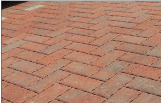
Permeable Paving - Public Parking Kilsaran Clima-Pave Slane - (Curragh Gold) Size: 200x100x80mm. Herringbone. Border: ClimaPave Newgrange. 3 Size Mix x 80mm in Black Granite. Soldier Course. (or similar approved)
