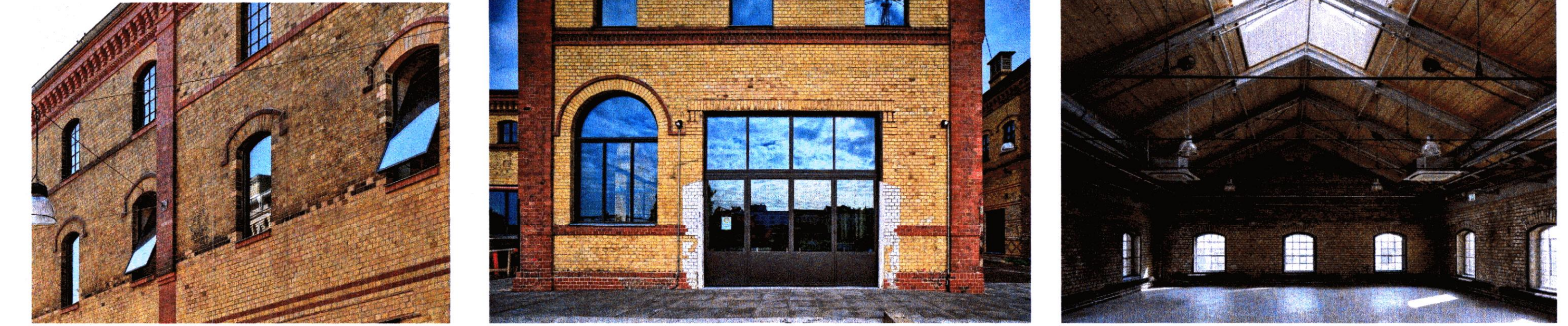
ALL PROPOSED GLAZING AND SECONDARY GLAZING DETAILS ARE BASED ON JANSEN JANISOL ARTE SYSTEM. REFERENCE IMAGES ARE SHOWING JANISOL ARTE SYSTEM USED IN HISTORIC APPLICATION
