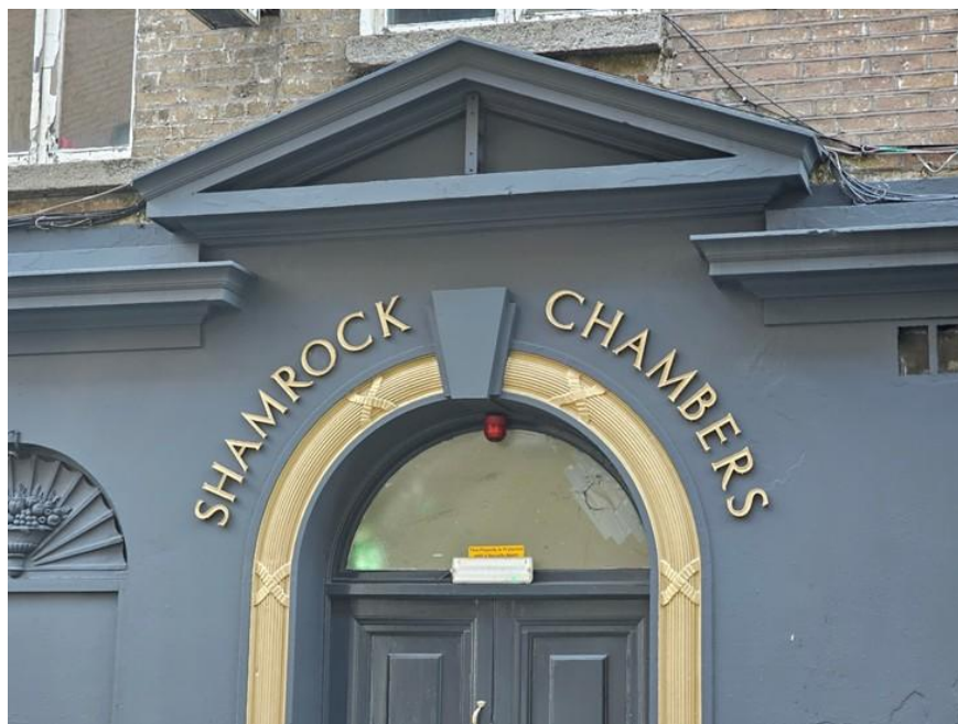
Plate 9: Detail of entrance to Shamrock Chambers
