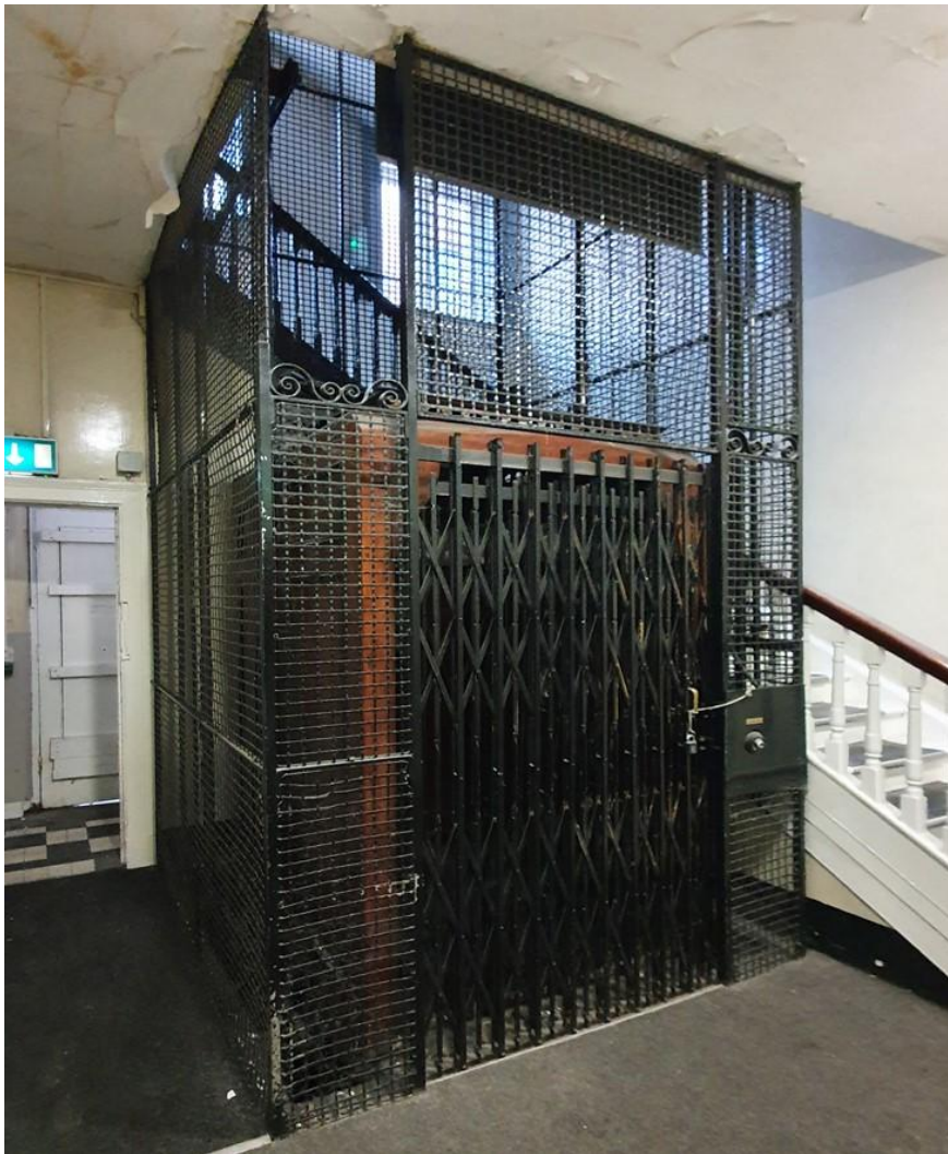
Plate 11: Cage lift at ground-floor level
