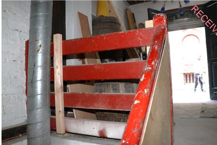
Plate 18: Staircase to basement
