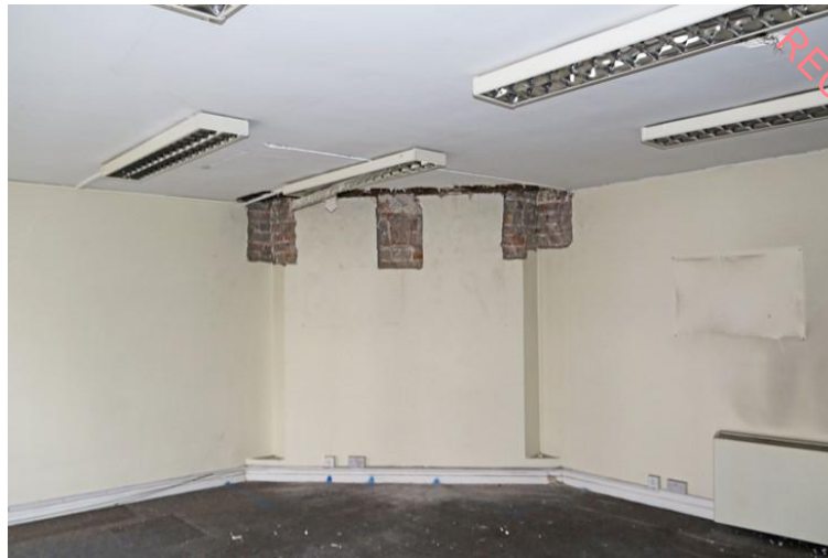
Plate 30: Corner chimneybreast in front room
