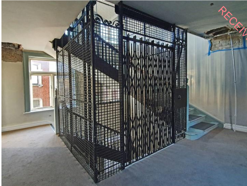
Plate 12: Lift cage at first-floor level
