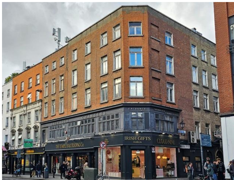
Plate 5: Corner view of Shamrock Chambers
